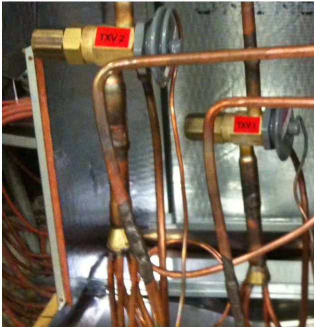
Thermal Expansion Valves
